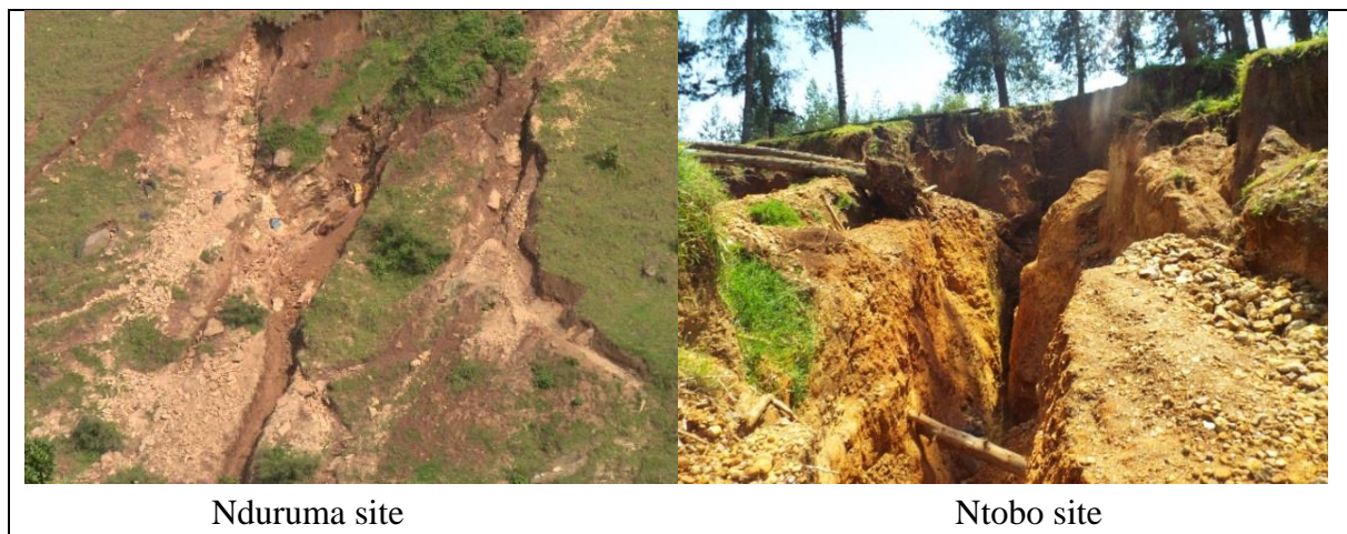
Figure 20: Photographs showing rills and gullies resulting from piping water
